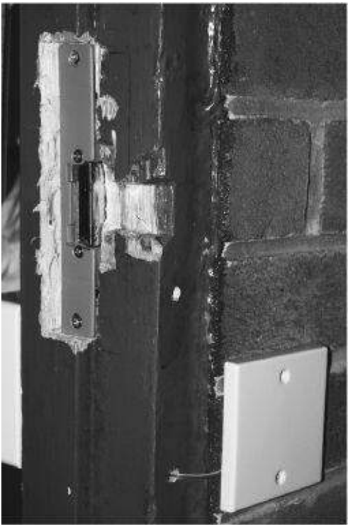
Figure 10-17 The RFID antenna installed outside the door
