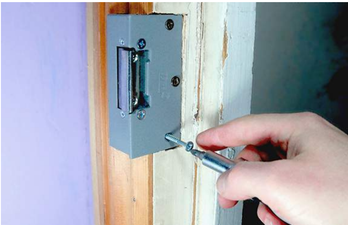
Figure 8-13: Installing the door strike.
