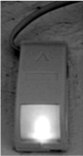
Figure 4-39. PIR sensor
