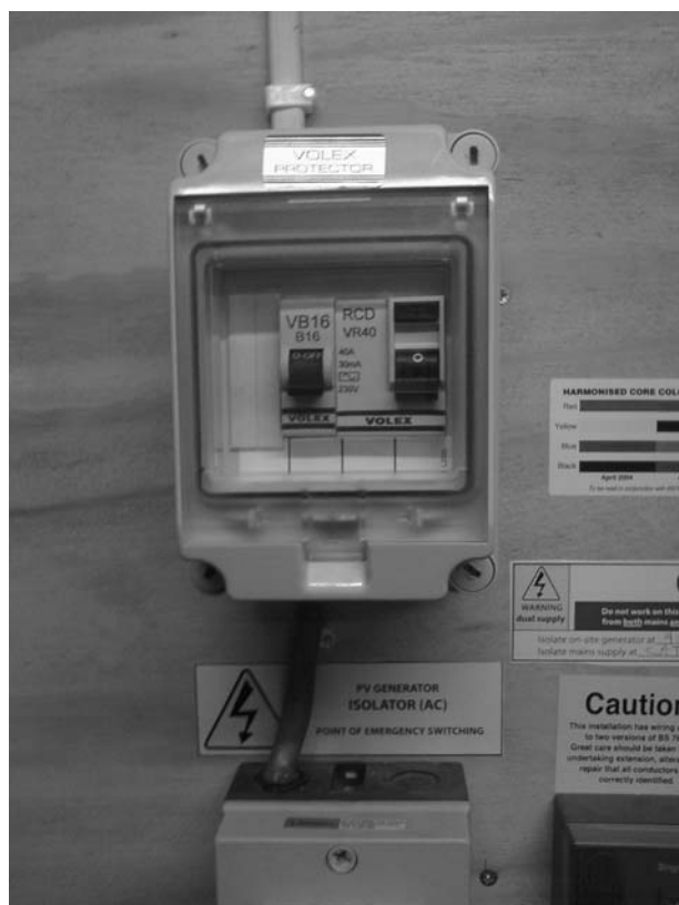
Figure 10-43 Mains circuit breaker.
