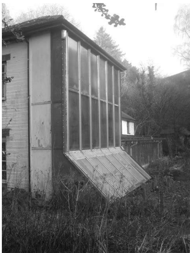
Figure 5-1 Trombe wall at CAT, U.K.
