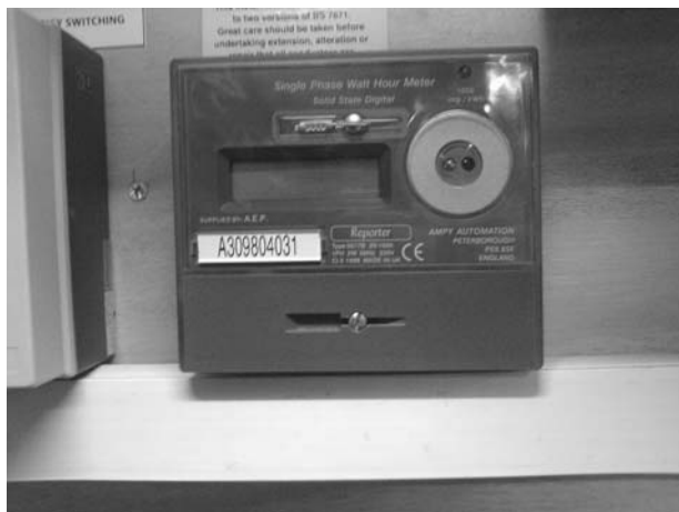
Figure 10-45 Watt hour meter.
