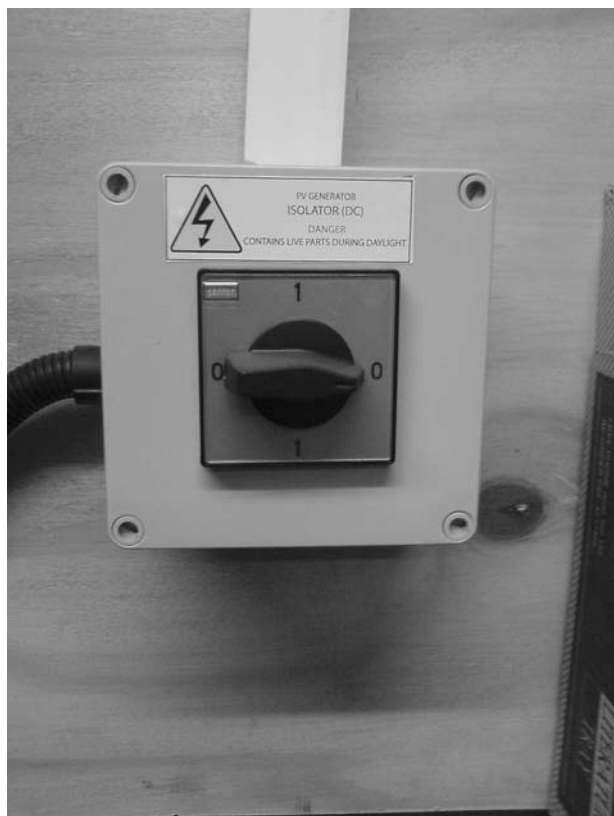
Figure 10-42 Mains isolator switch.
