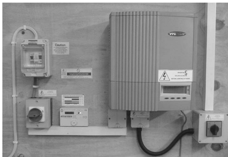
Figure 10-41 A typical inverter setup.
